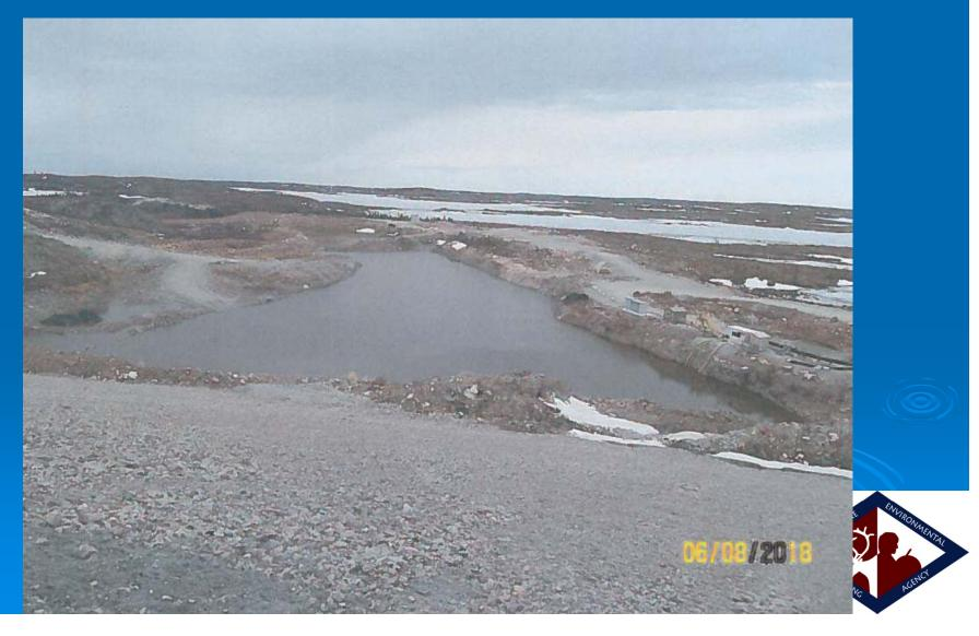
Day Tank 2 (spill 17-440 spill site): staining on the ground indicates the extent to which diesel overtopped the sump and infiltrated the ground. De Beers will remove this material soon
