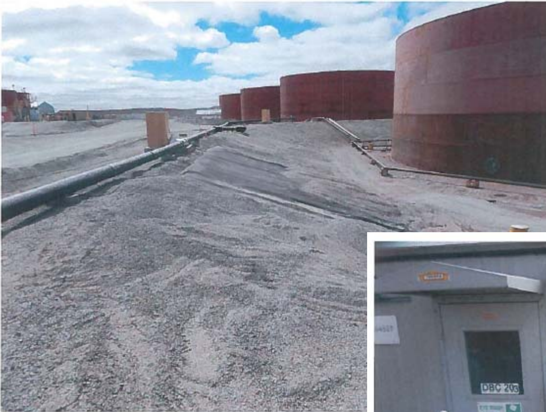
Photo 8 – 10 Million Liter Tank Farm – The containment area was dry and no concrete tank farm will need to be covered as per the liner design.
