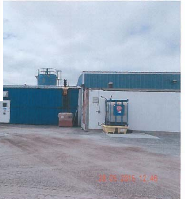
Photo 32 – Emulsion Plant – The area around the Emulsion Plant and the offloading point for Ammonium Nitrate were clean with no evidence of spillage.
