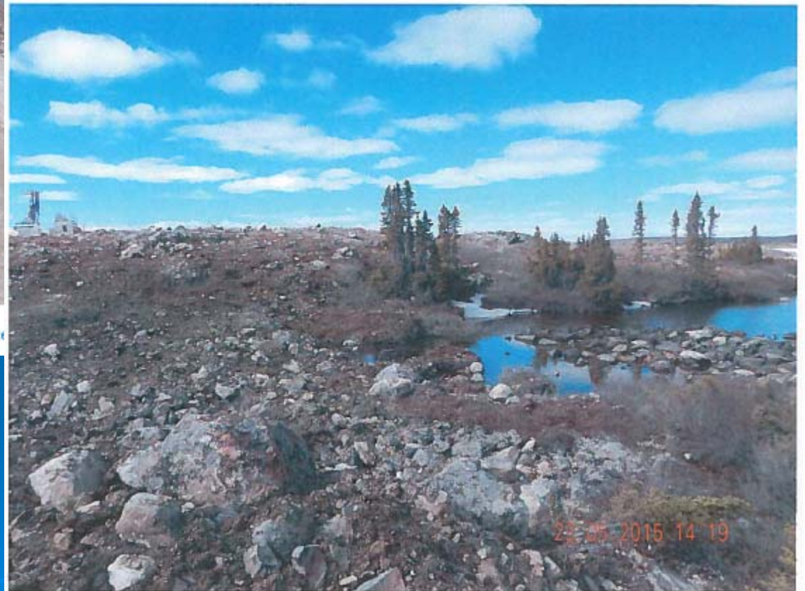
Photo 34 – North Pile West Cell – Organic soil removed from the West Cell Tote Road and grout curtain construction area had been placed within close proximity (<30m) of Snap Lake. The soil has since been removed and placed at the former AN storage pad to be used for reclamation research. Inspection showed that the soil did not get placed into the lake and there is no damage to the tundra underneath.
